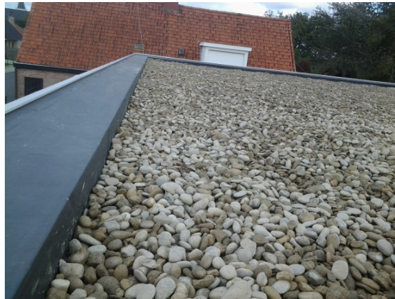
Foto dakplatform in EPDM ter illustratie
